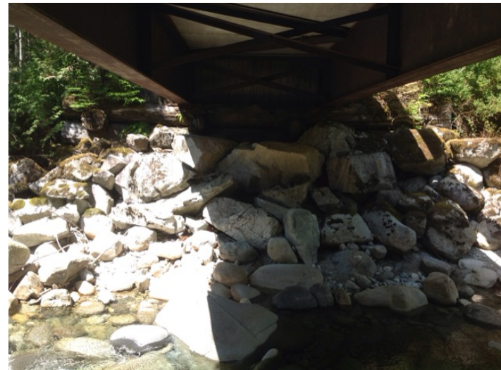
Right Bank Abutment when facing downstream
