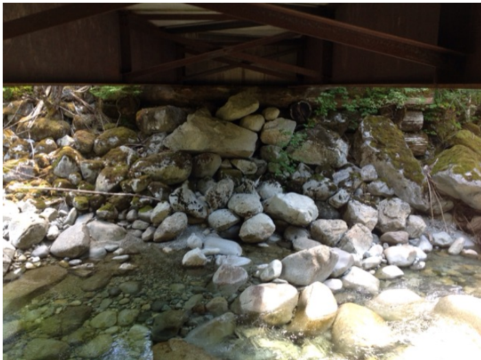
Left Bank Abutment when facing downstream
